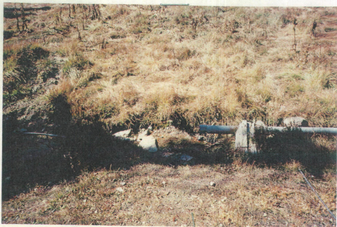
Pipe coming from Spring
