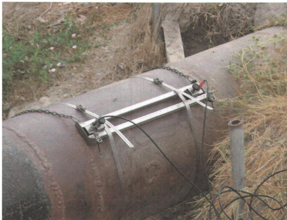
Elijah Drain Transducer Installation
