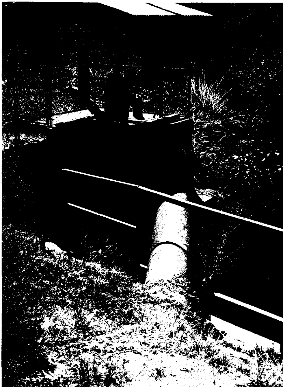
Elijah Drain Pump and Discharge Pipe
