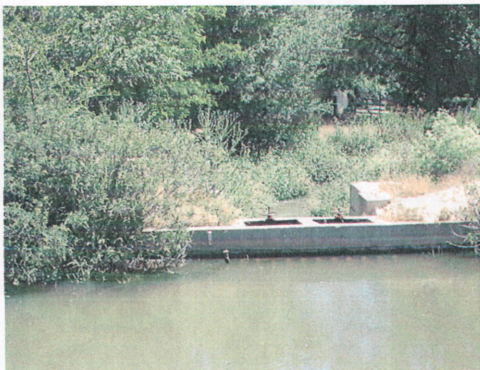
The Campbell Canal diversion.
