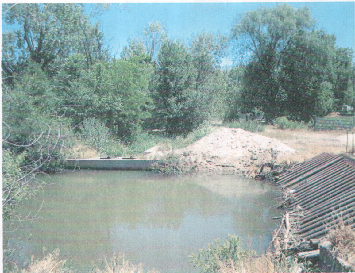
← Sebree Canal diversion
