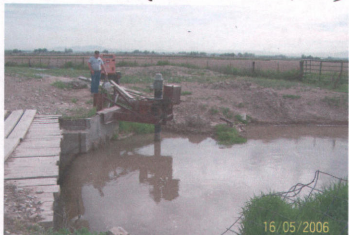
Riverside Canal supplemental water intake 5/16/06
