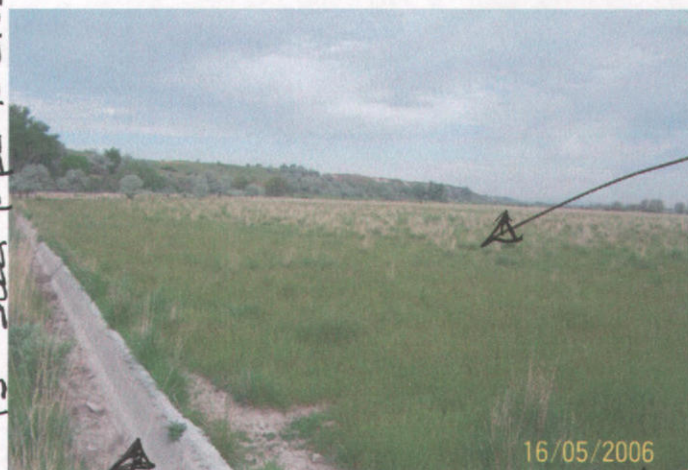
15" steel pipe to cross Canal 5/16/2006 SH
