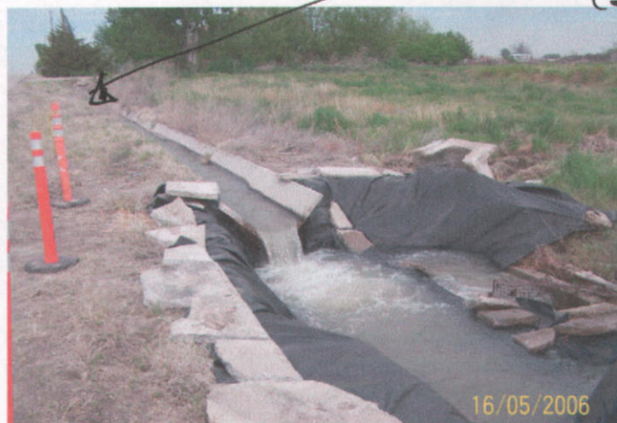
POD: Wastewater 5/16/06 SH
