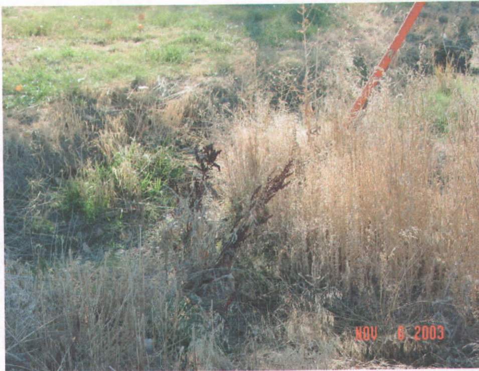
Ditch onto property from POD #2 facing W.
