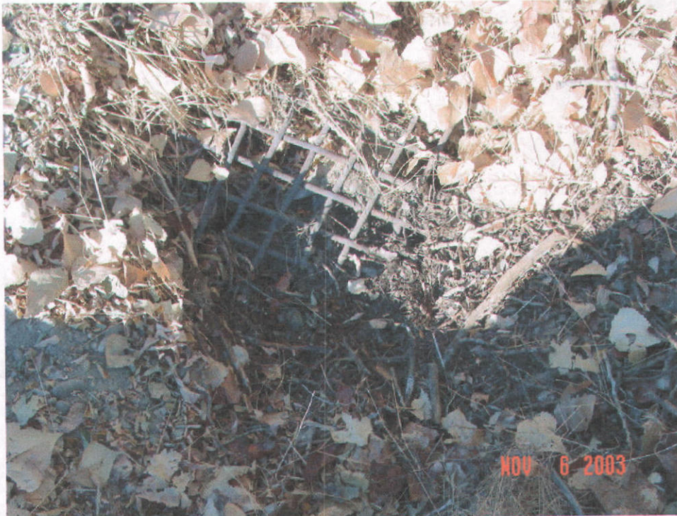
POD #2 Catch drain to collect wastewater across road from house.
