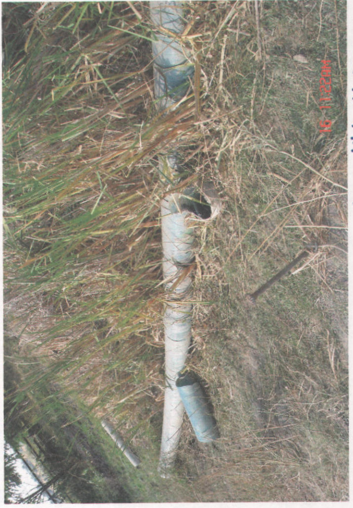
replacing feed ditch w/ pipe
