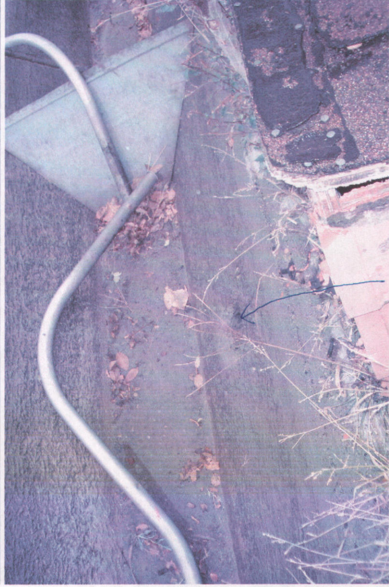
Pic#2 Cement ditch with inlet From pump
