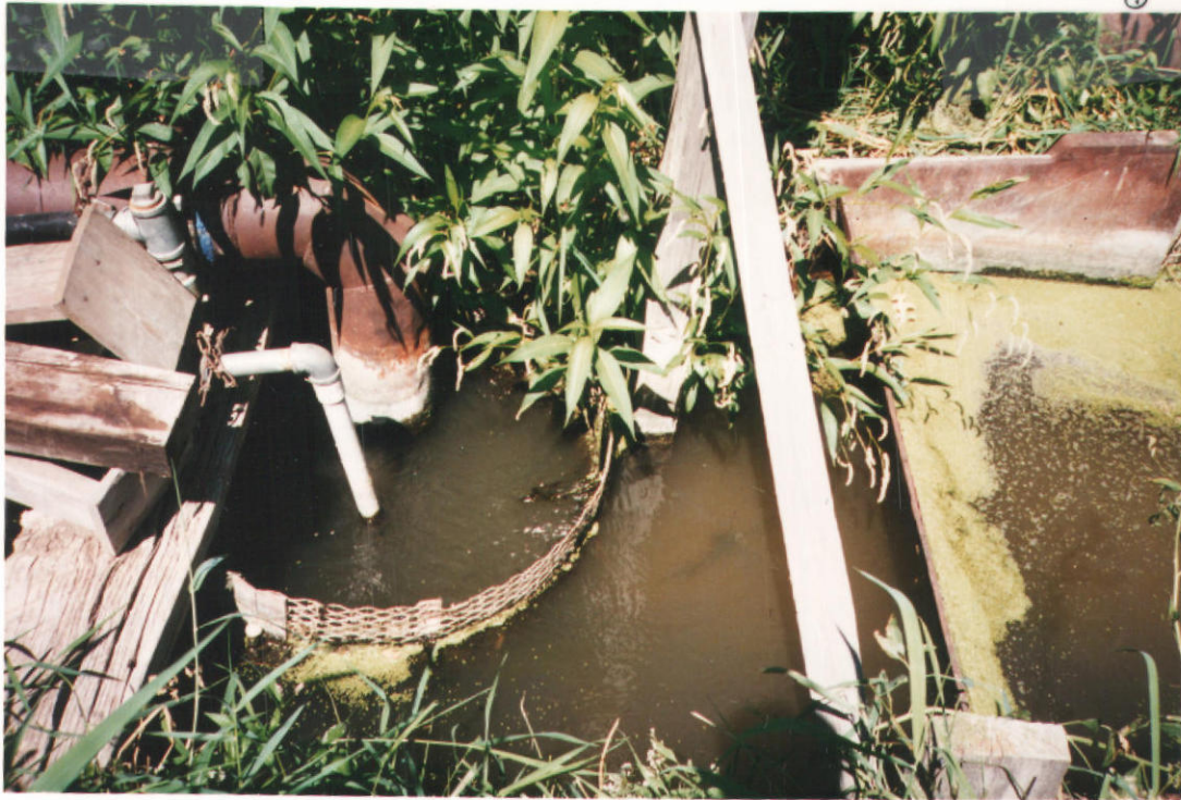
① Intake from Scott Drain. SESWNE On North side of Boulder Lane, on west bank of Scott Drain.
