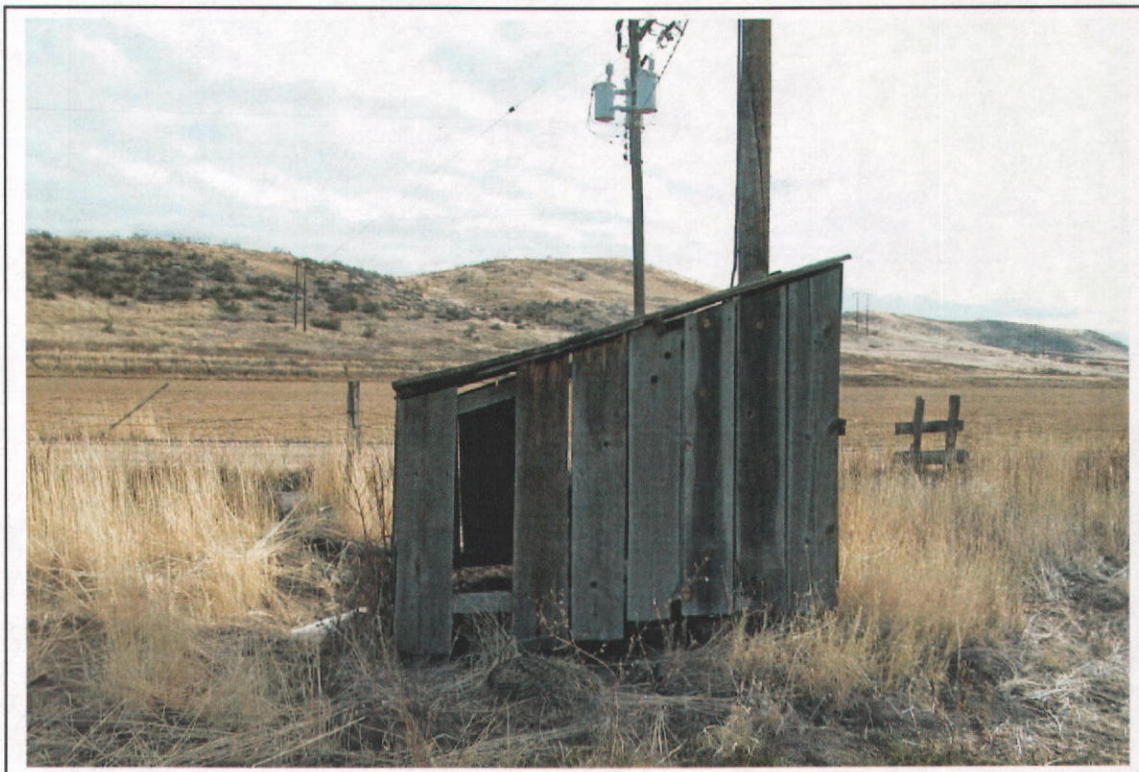
Photo 2: Well house. View is to east. New system from well delivers water in underground piping into a distribution pond where the groundwater is commingled with Dry Creek water. Re-lift pumps put water in to a pressurized underground sprinkler system. See attached Enchanove Ranch Estates plats for detailed irrigation system.
