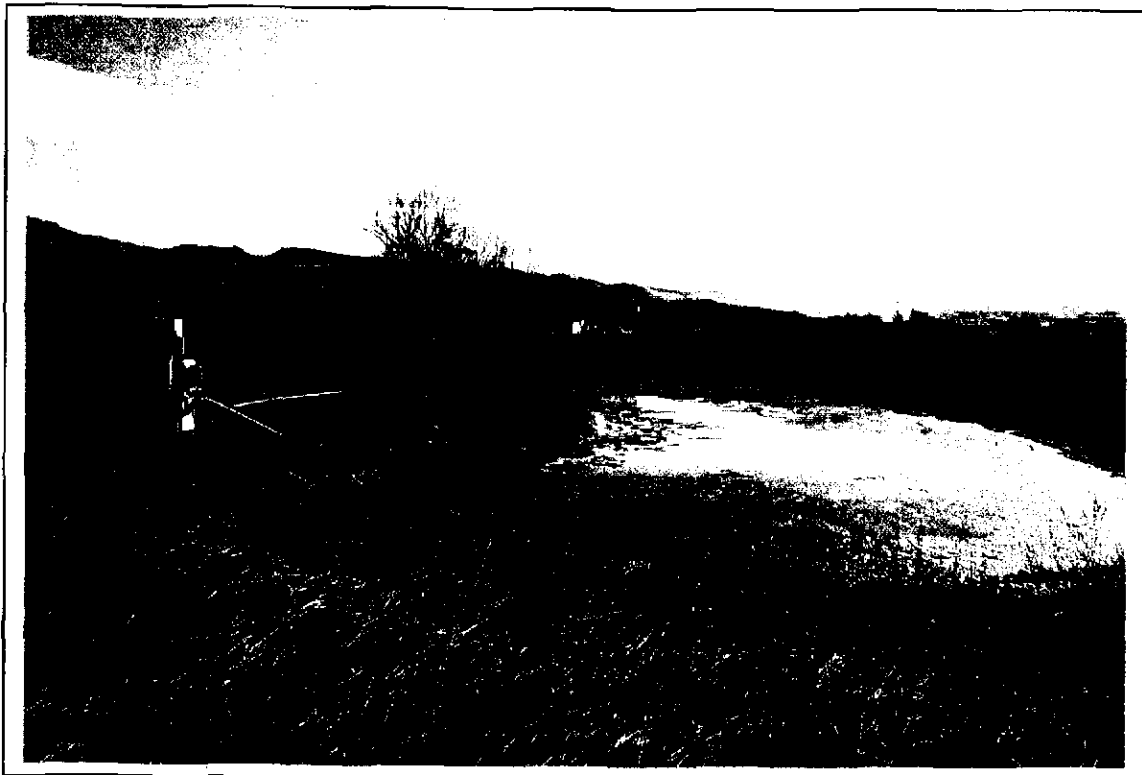
Photo 4: Distribution pond & pressurized system, view is to the east. See attached measurements. The pond has 5.17 AFA volume MAX. The well water is supplemental to surface Dry Creek right and thus the MAX combined flow is 2.78 CFS. (2.78)(1.9835) = 5.51 AFA.
