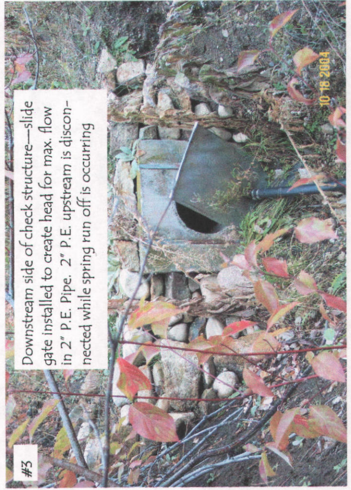
2" P.E. pipe goes to farmstead for irrigation.
