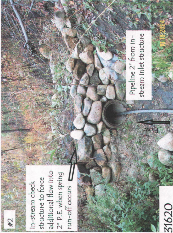
In-stream inlet structure
