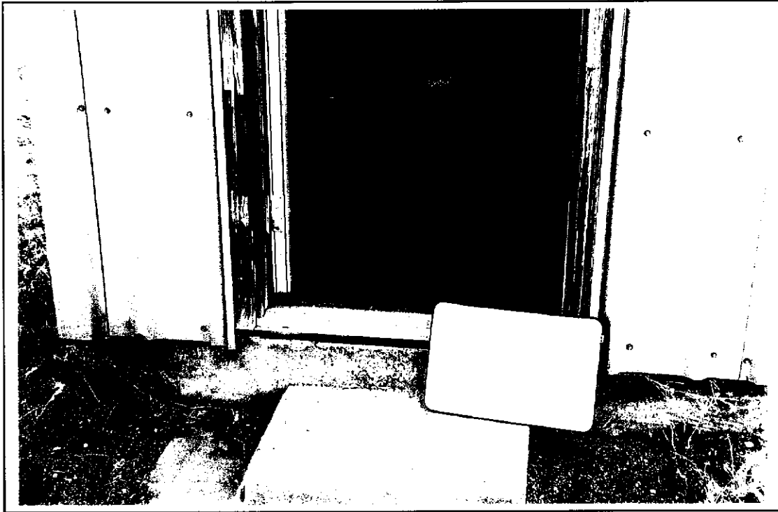
Photo 3. Well house, point of diversion located in the NWNESE, T05N, 02E, S28.
