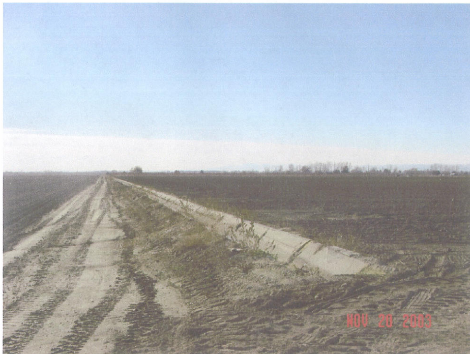
Ditch facing south from 4 corners re-diversion point
