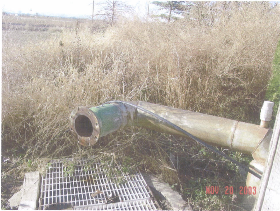
POD where pump would sit to draw water from pond facing W.
