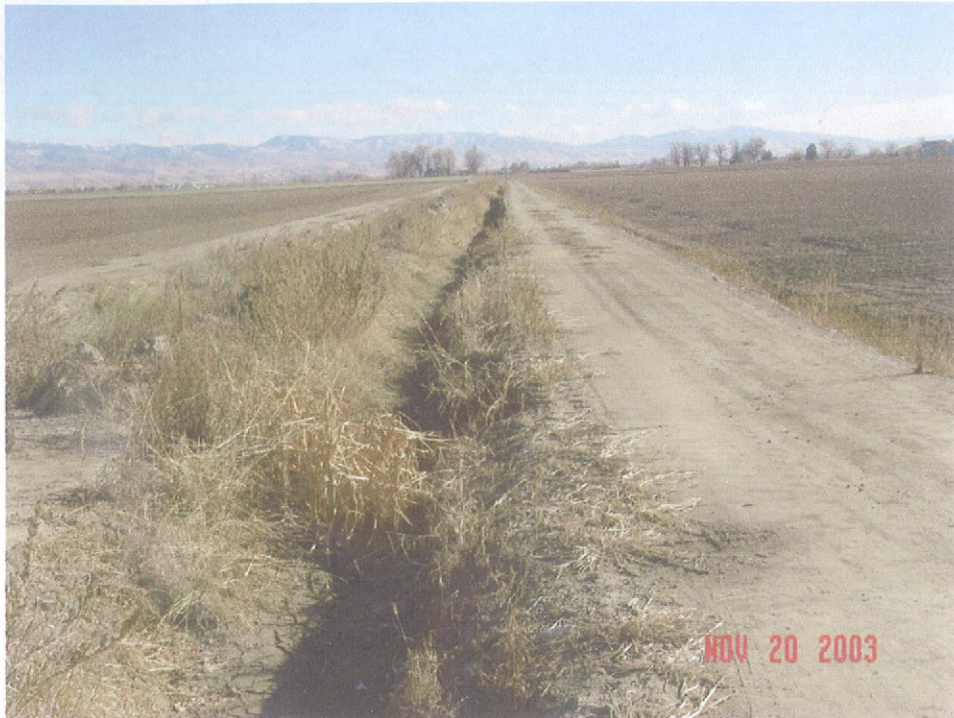
Ditch facing east from 4 corners re-diversion point
