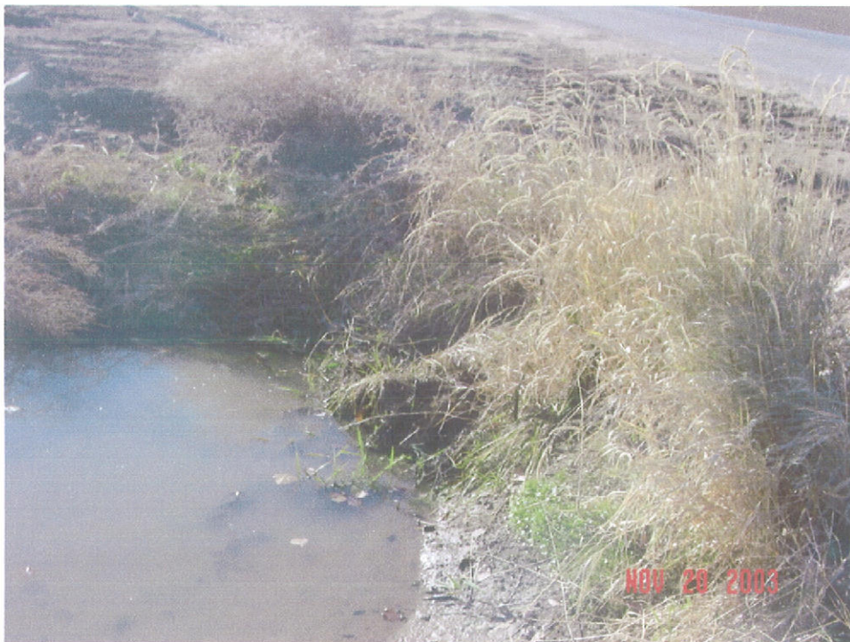
Drain pipe at west end of pond
