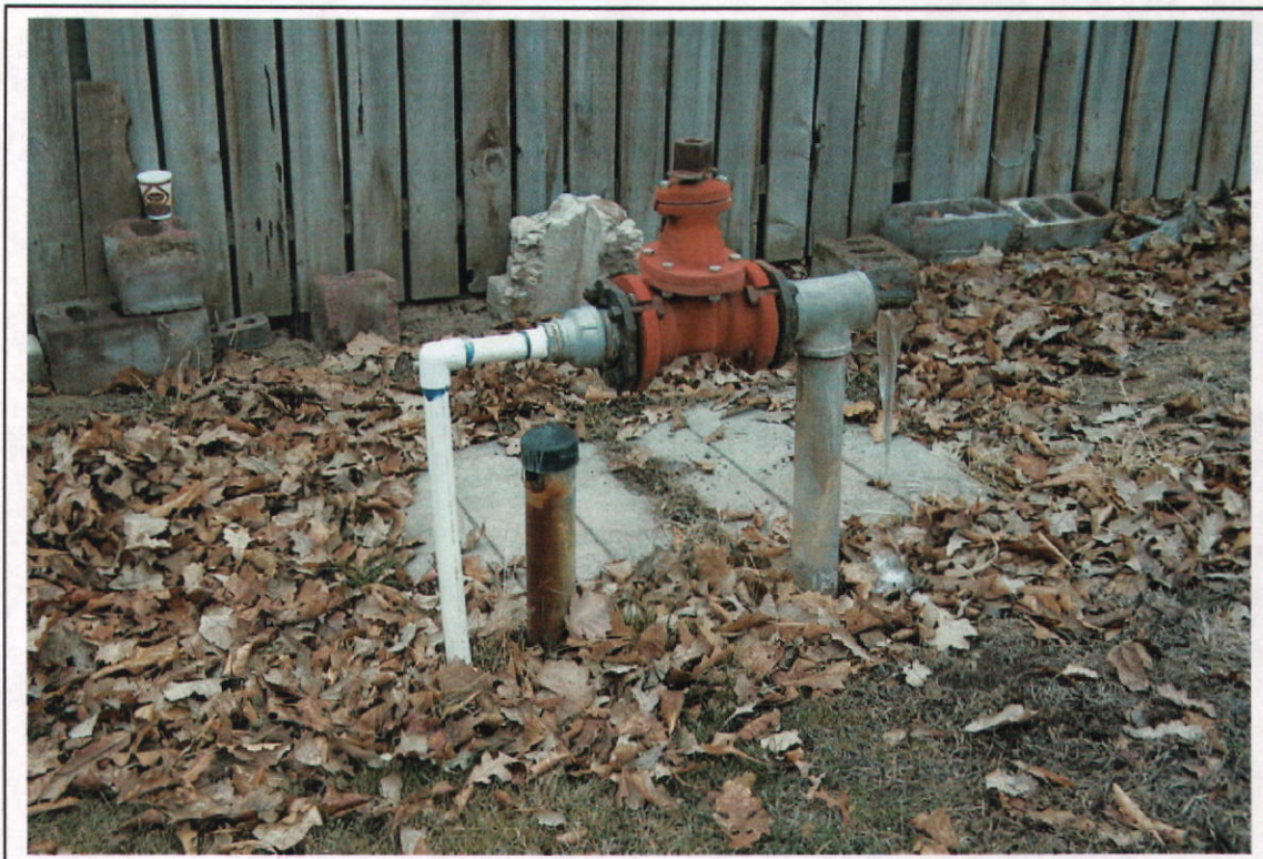
Photo 1: 63-24140, Field Exam 01-09-03: Located in the SESWSW, S08, T04N, R01W. This is an artesian well with 4 inch casing. No pump. Closed system.
