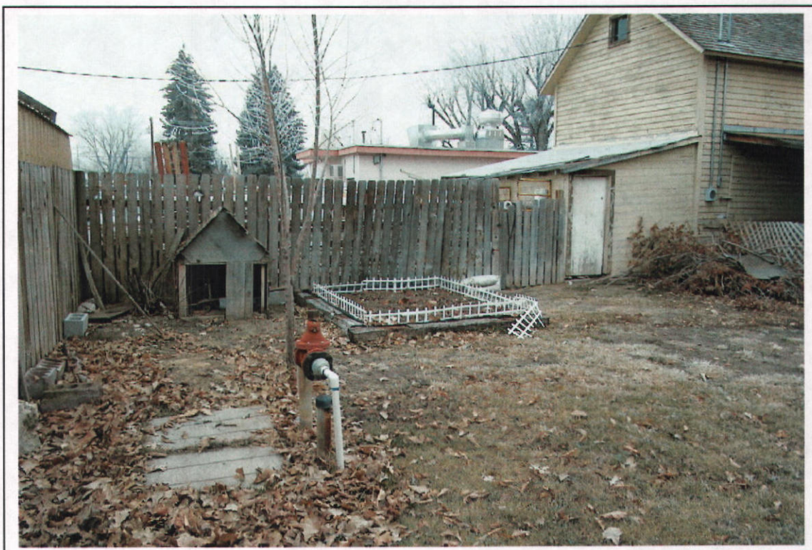
Photo 2: Same well. View is to west. Old system delivers water into store heat exchangers and 2 bathrooms. Underground piping to store, then injects cooling water used for cooling into injection well. Restroom wastewater is not injected. Photos by RDH.
