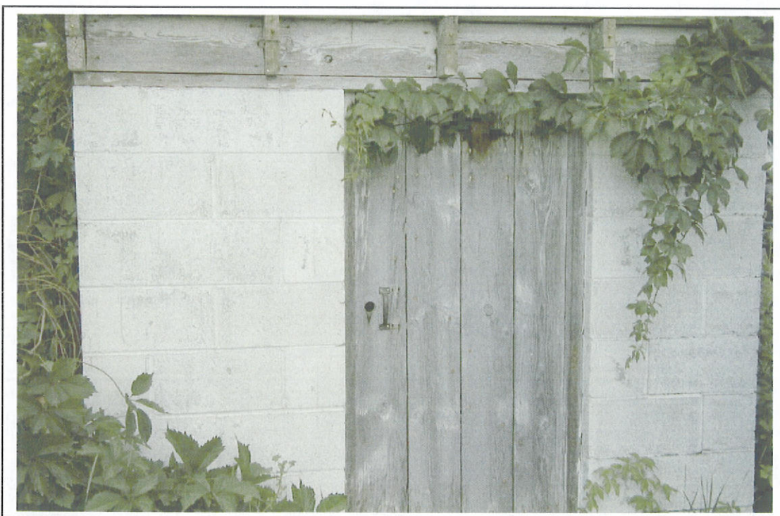
Photo 2. Outside view of well house. Located in the SWSE, T03N, R02E, S11. Water is piped underground to the east to the re-lift pumps about 150 feet.
