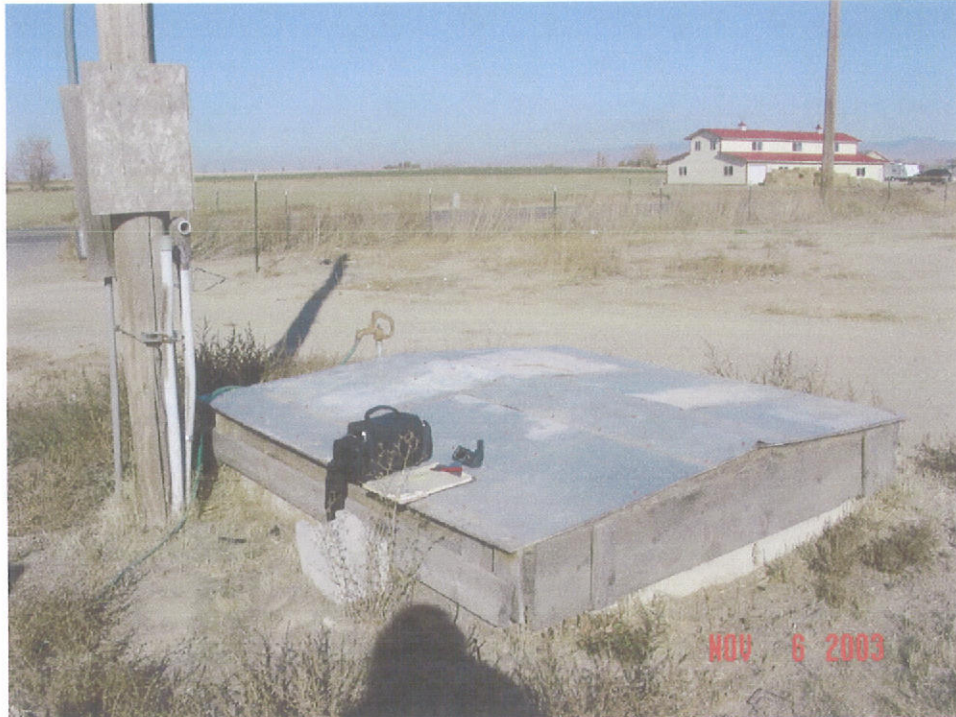
Well location facing NE.
