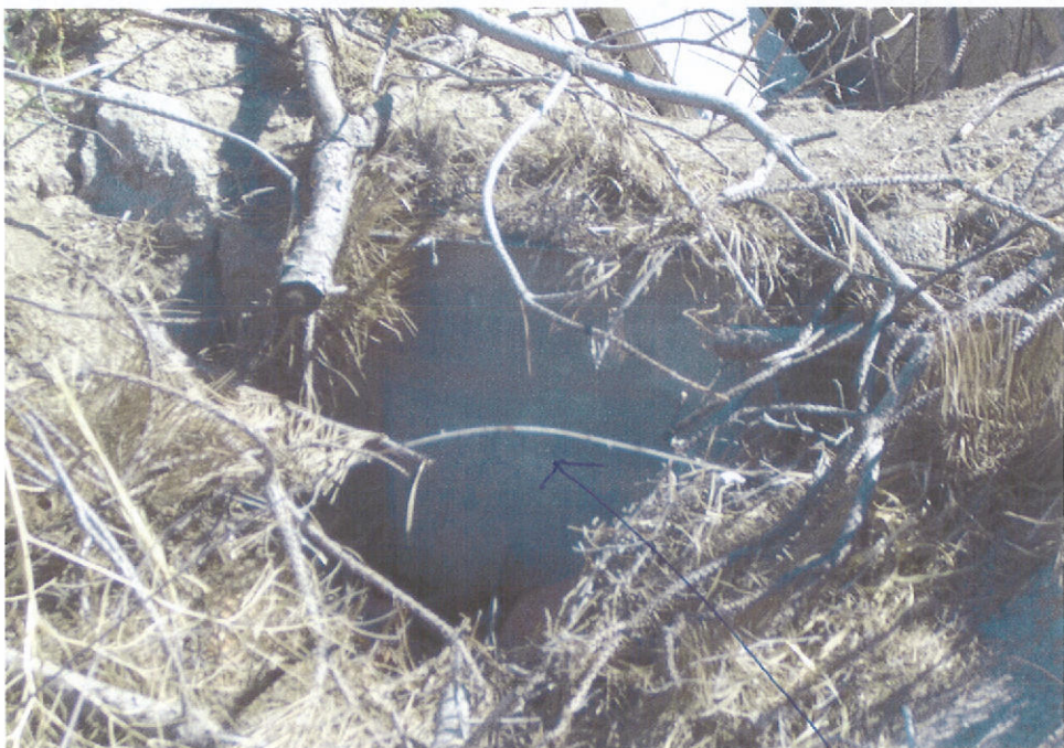
Picture # 28 30 GPS 2314611 12" slide gate USR 1395323 @ Head of Diversion
