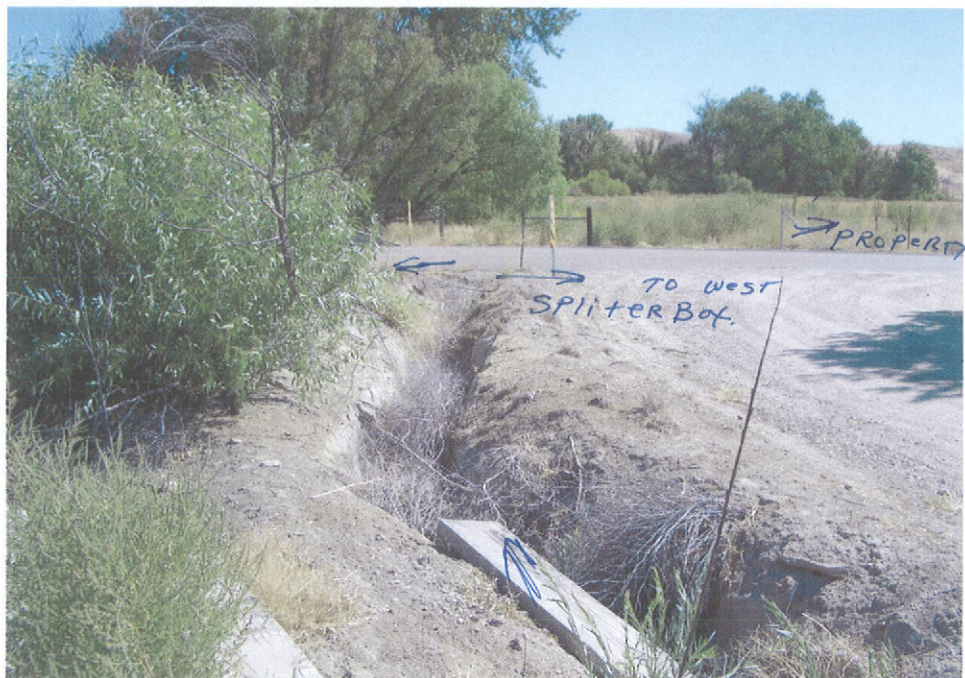
Picture # 28 31 Water Flow below Diversion point (15')
