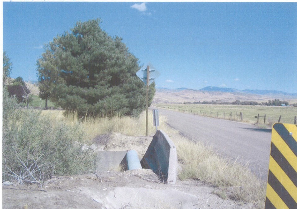
PIPE ACROSS SPRING CREEK TO THE EAST
