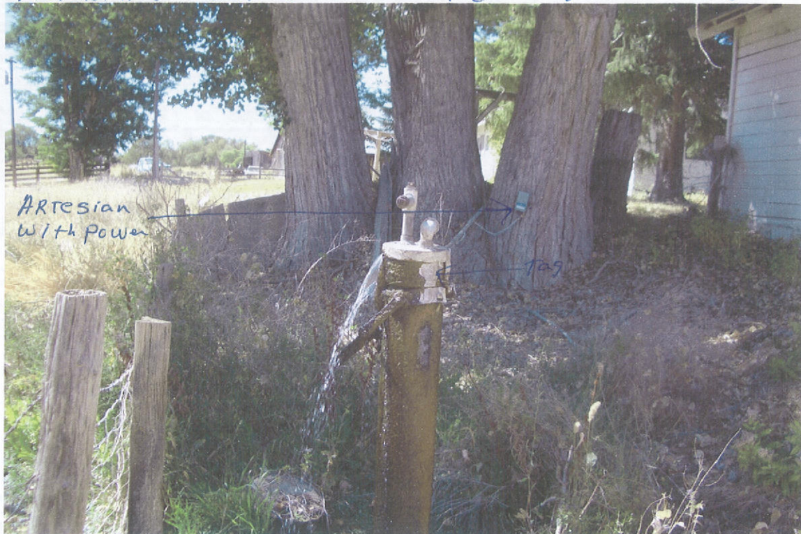
Picture # 12 Artesian Well By Existing House Tag on well Not Legible.
