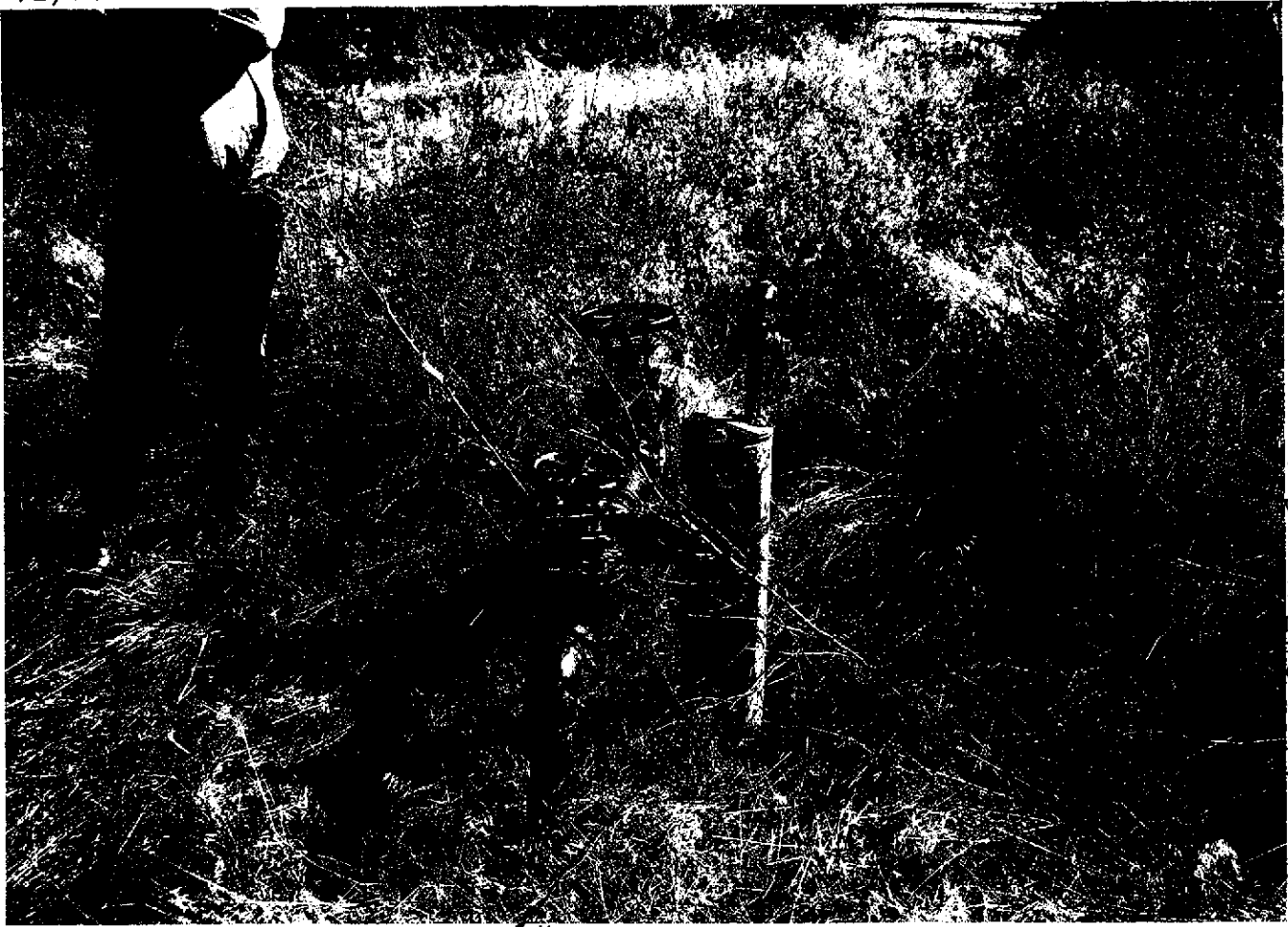
6" Well casing, with 4" lines to feeder ditch
