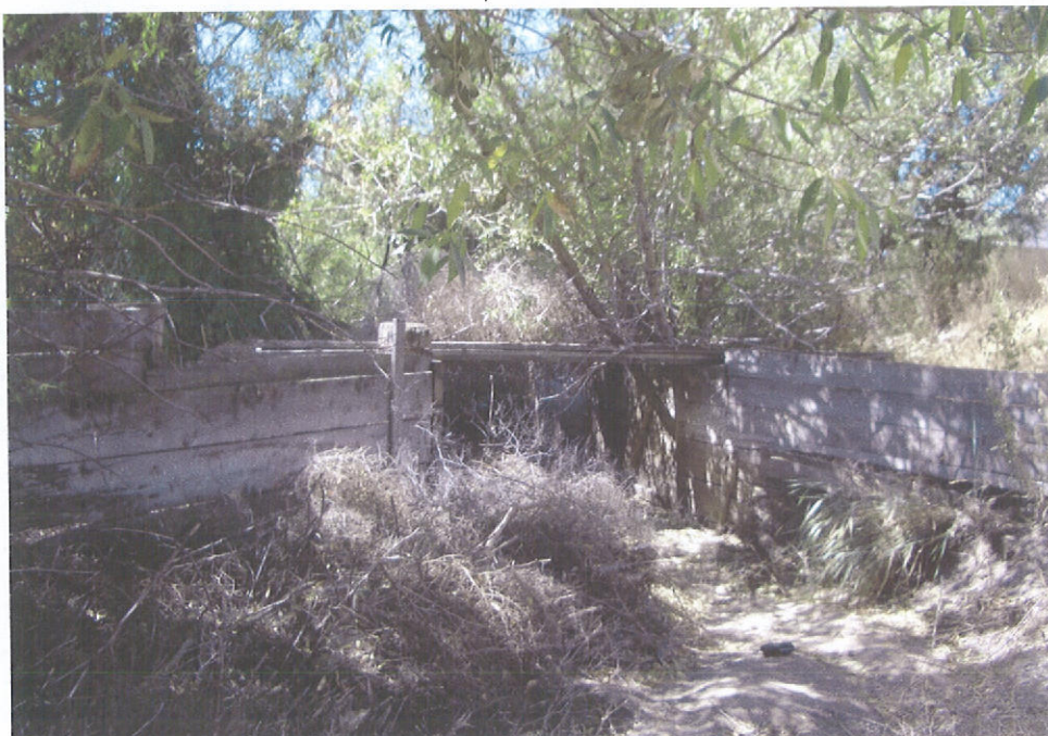
Picture # 3 Check structure in DRY CREEK. GPS. 2317410 4' W X 6' Wide USR. 1394855
