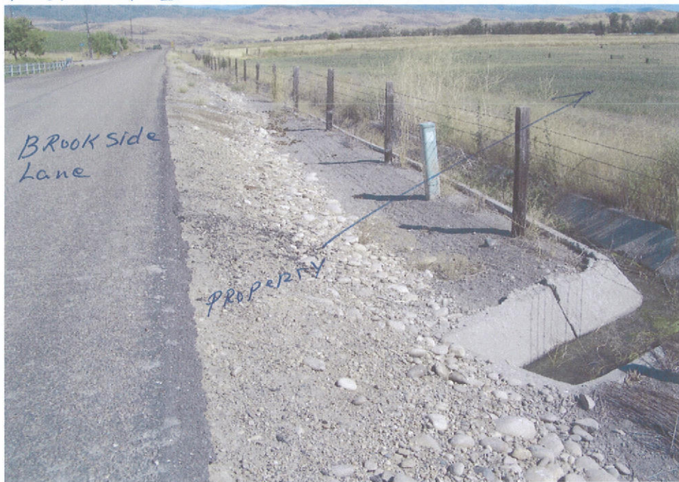
South Side of Brook Side Lane, Out let to Cement ditch See Pic. # 35 for Head of crossing
