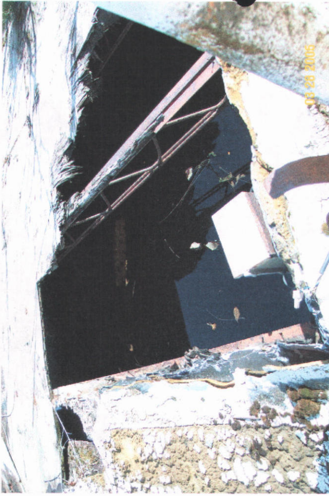
Top of Storage Tank
