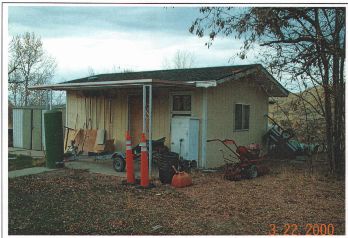
Photo 3: Photo by Intrepid Engineering Services showing well house.
