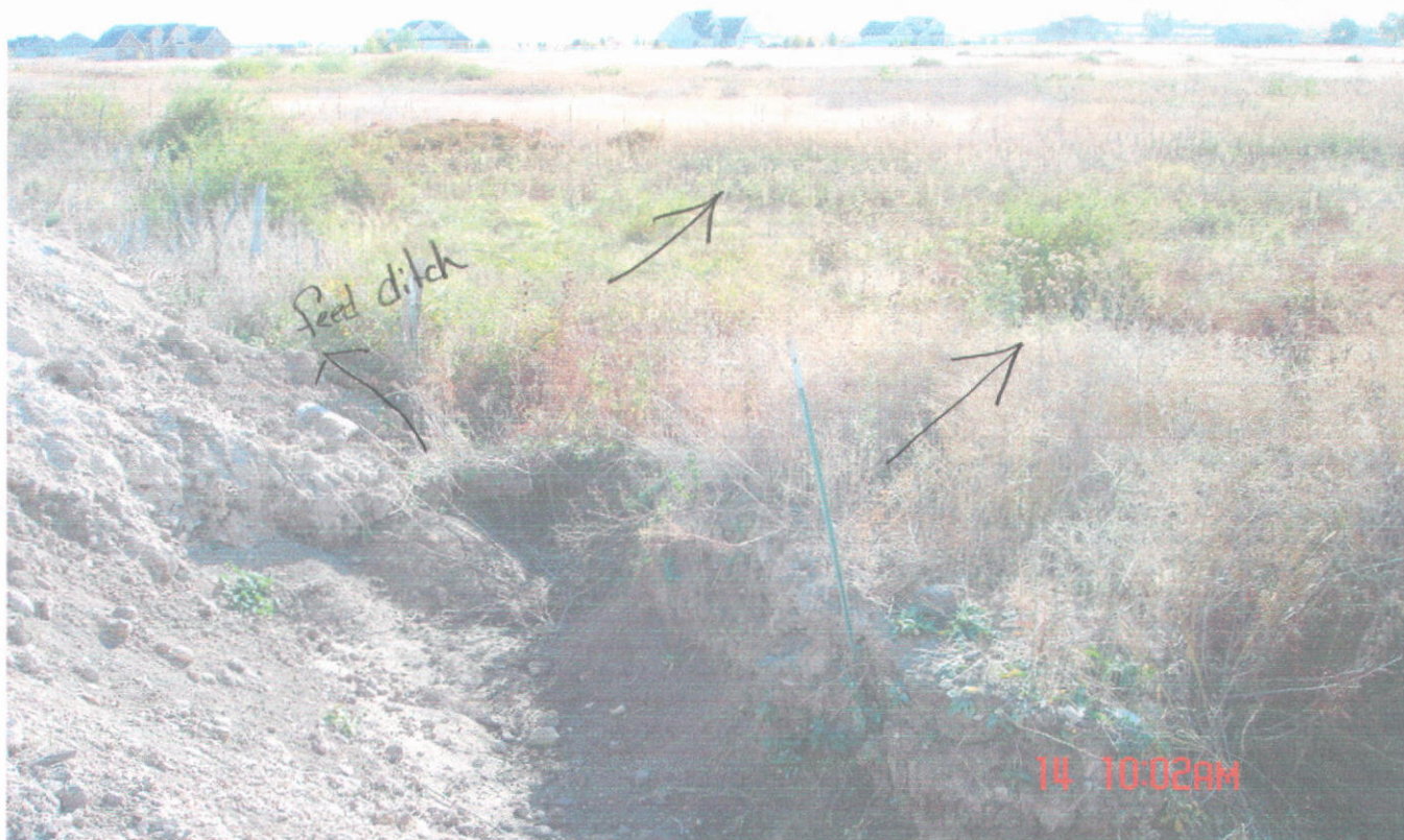
3rd Pod Pipe was being worked on.
