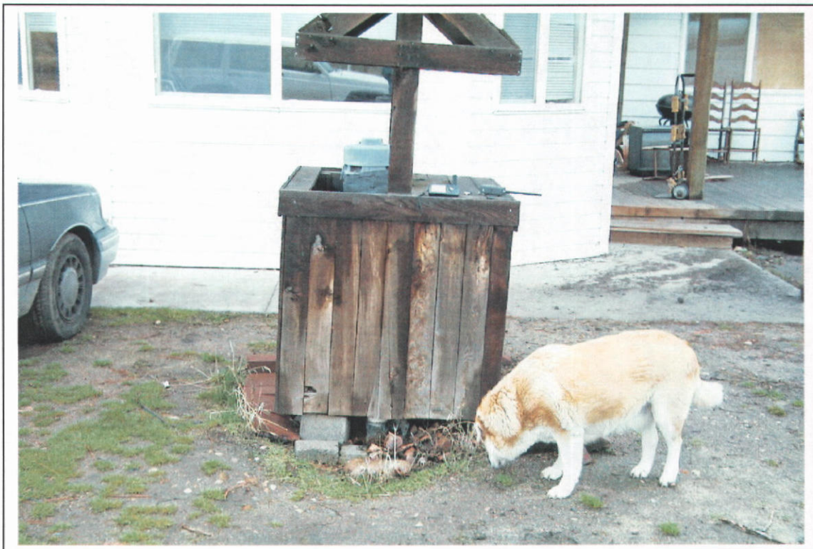
Photo 4: Irrigation well. Sprinkler systems, hand lines, 40 HP pump, 55 PSI per owner. Static water level measured at average of 53 ft. See attachments. Photos by RDH.
