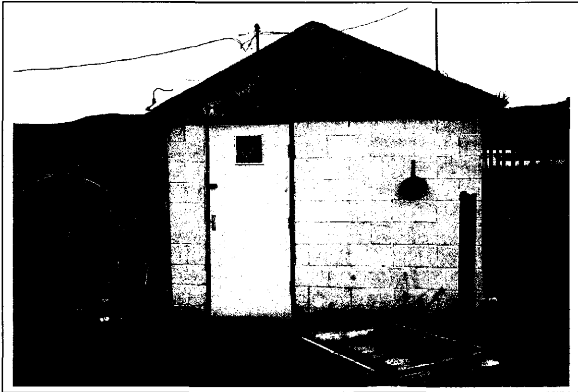
Photo 3: Outside of the Domestic well house. View is to North.
