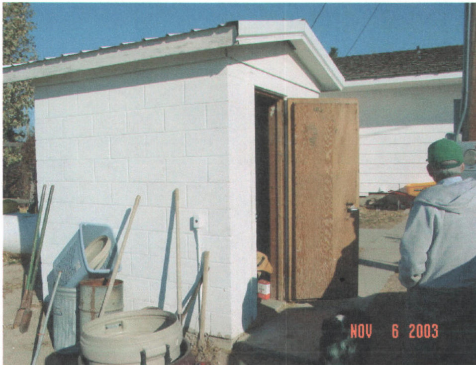
Pump house facing East.
