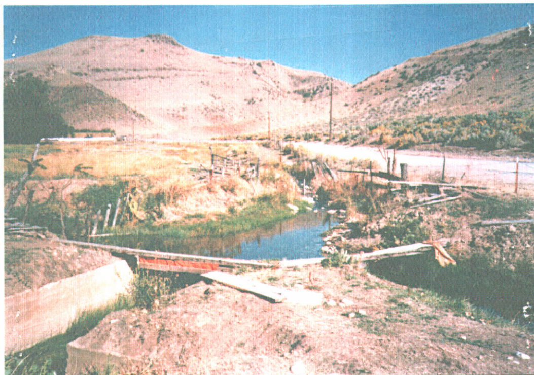
Rediversion point B where Warm Springs Creek intersects the Penitentiary Canal
