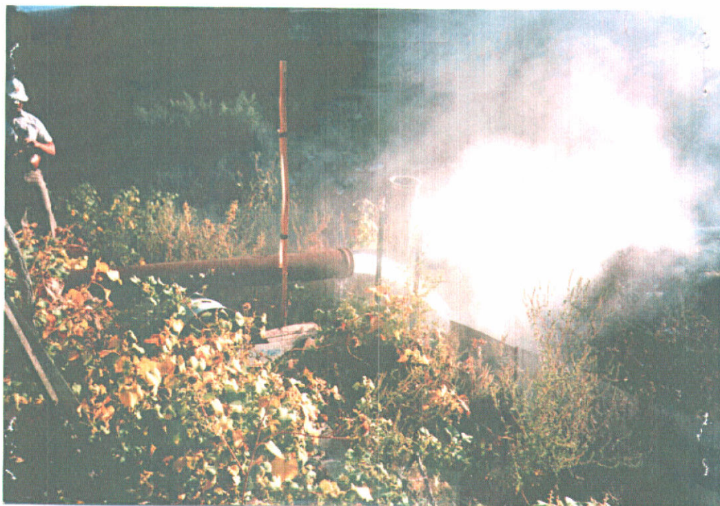
Looking North- northeast at discharge pipe with orifice plate attached.
