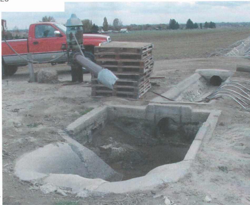
WELL AND CONCRETE DITCHES
