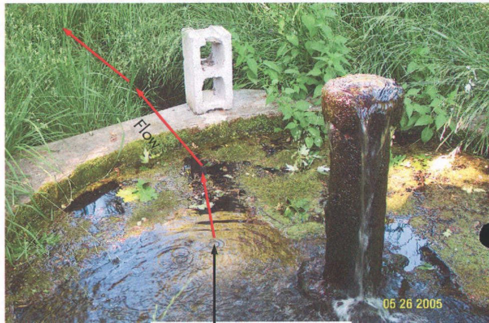
Water Flow into ditch
