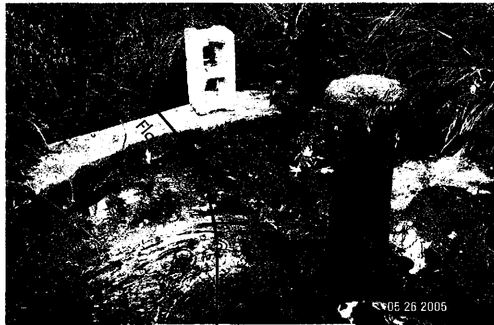
Water Flow into ditch
