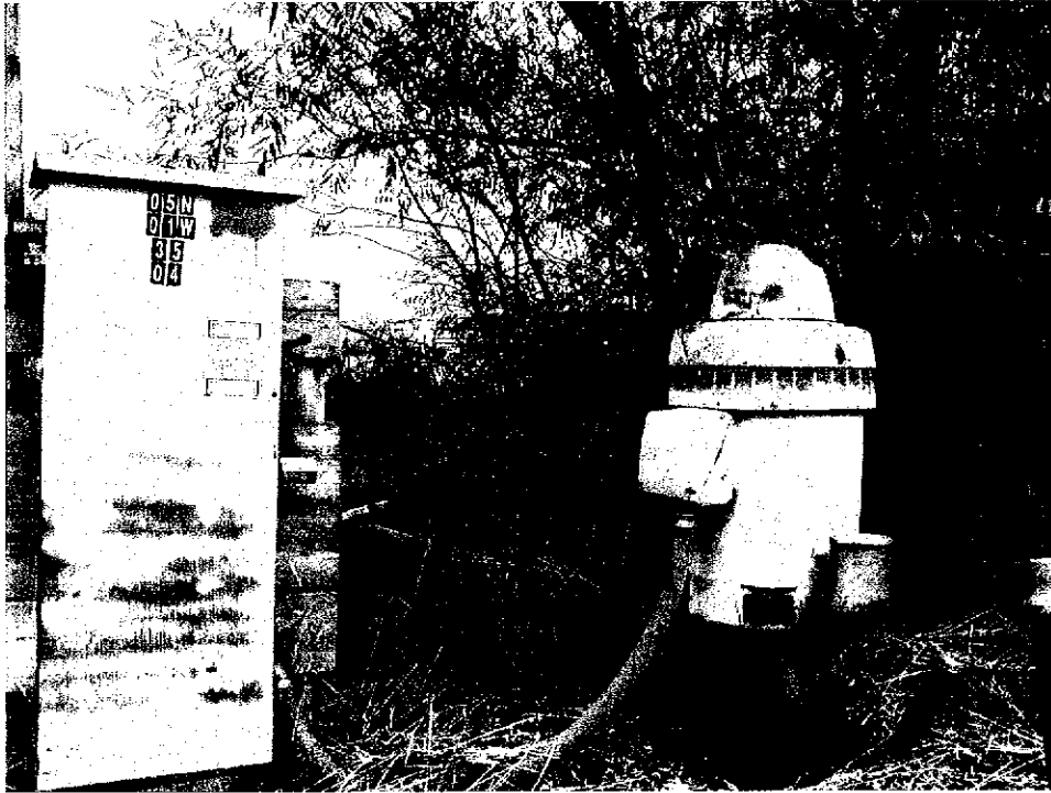
Pumping system facing NW.
