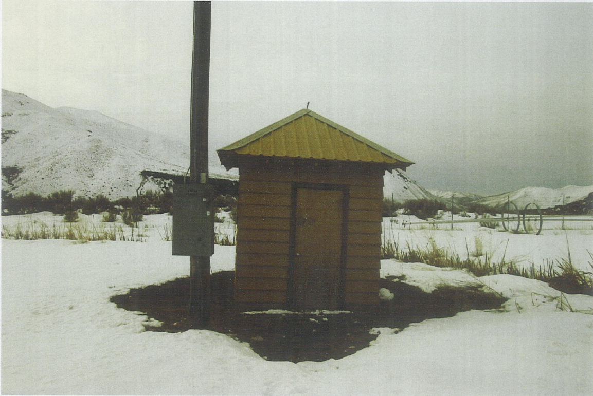
Looking South. Pump house that holds domestic and commercial well (csaxton 2/13/02).
