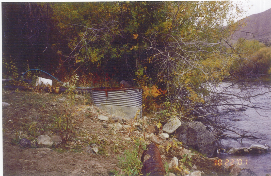
PHOTO # 1 LOWER POINT OF DIVERSION AT THE 20HP PUMP & MOTOR
