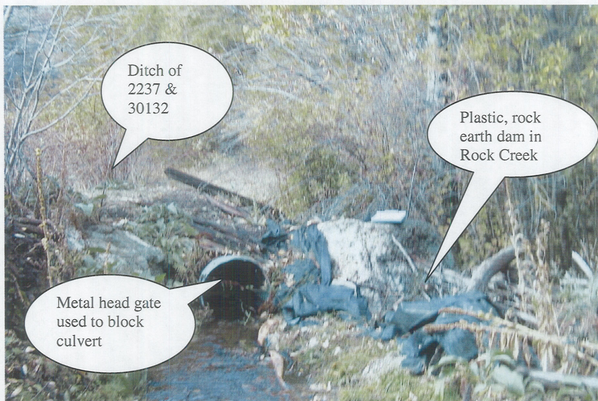
Photo 1. FX Oct. 11, 2001. Photos by RDH. POD Rock Creek for 63-30132 overlap with 63-2237 GPS location, T01N, R08E, S07, NESESW.
