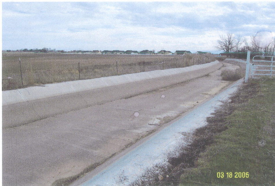
From Canal Bank looking Southeast
