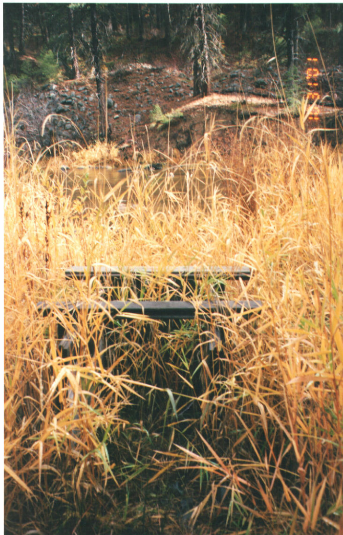
PHOTO # 10 POINT OF DIVERSION AND DIVERSION STRUCTURE IN THE SESW, S35, T6N, R4E.
