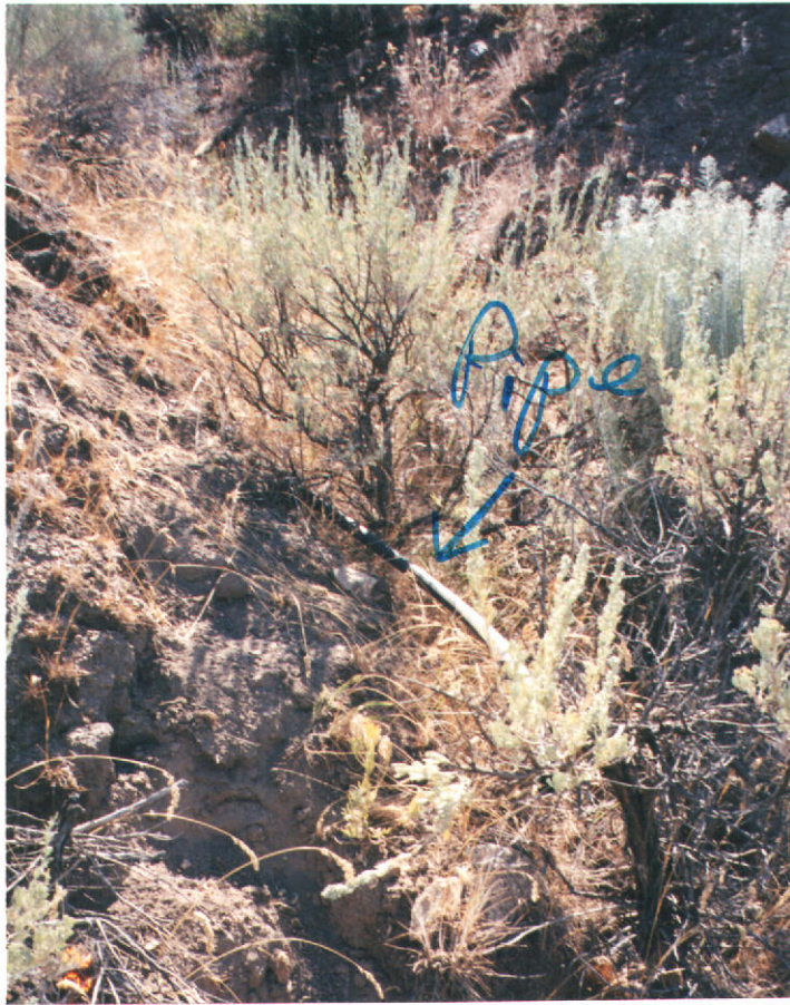
PHOTO #5 PIPE FROM UPPER SPRING
