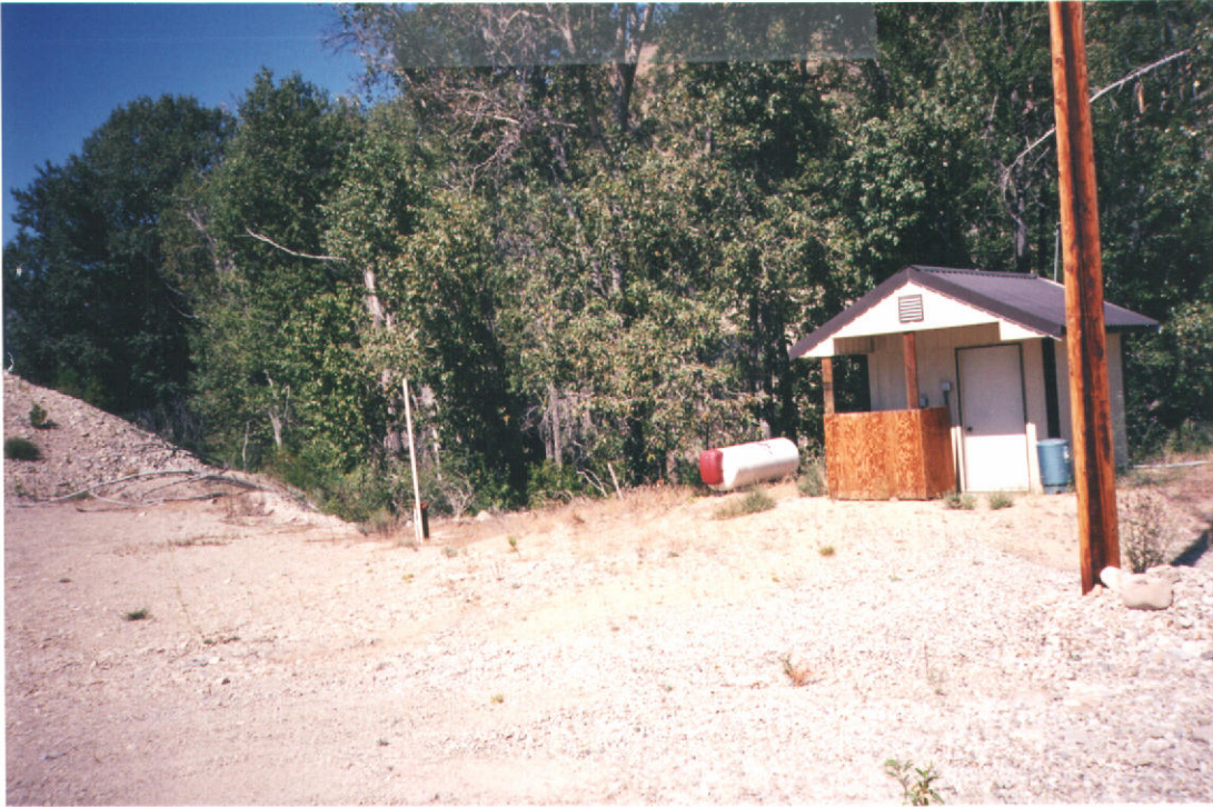
Well #1 located to the S.E. of Wellhouse
