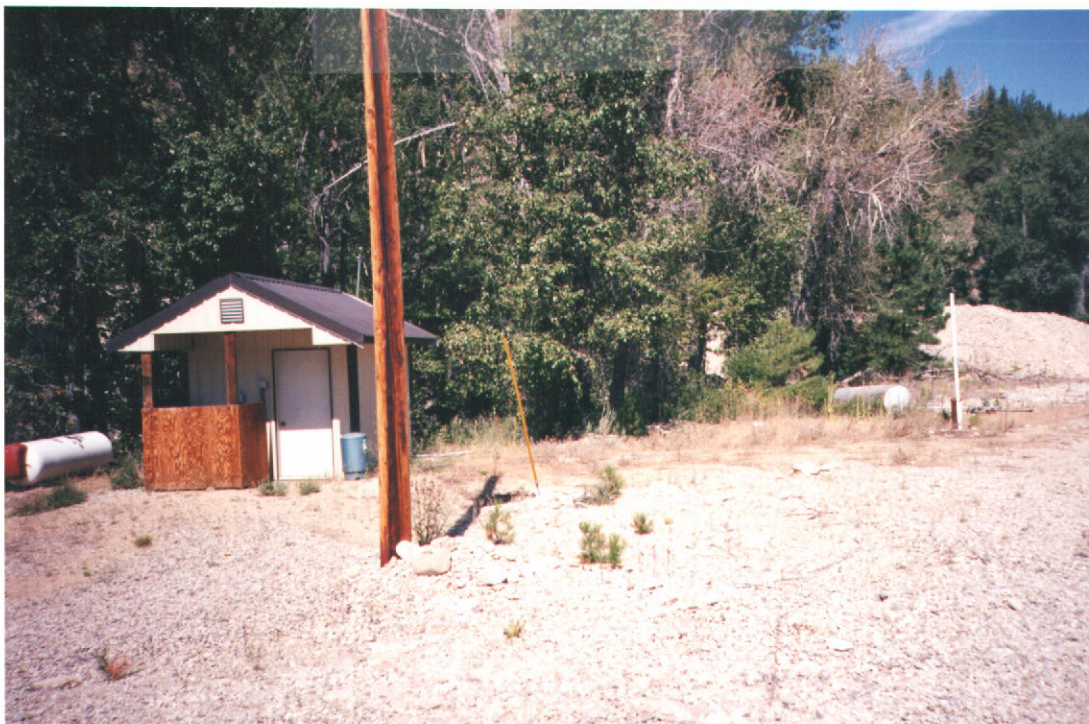
Well #2 located to the N.W. of Wellhouse
