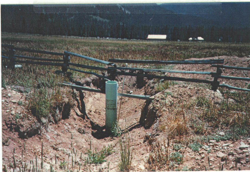
RISER AT EDGE OF PASTURE. FIELD IS FLOOD IRRIGATED IF NECESSARY. WORK ON RISER CONTROL VALVE WAS REASON FOR EXCAVATION.
