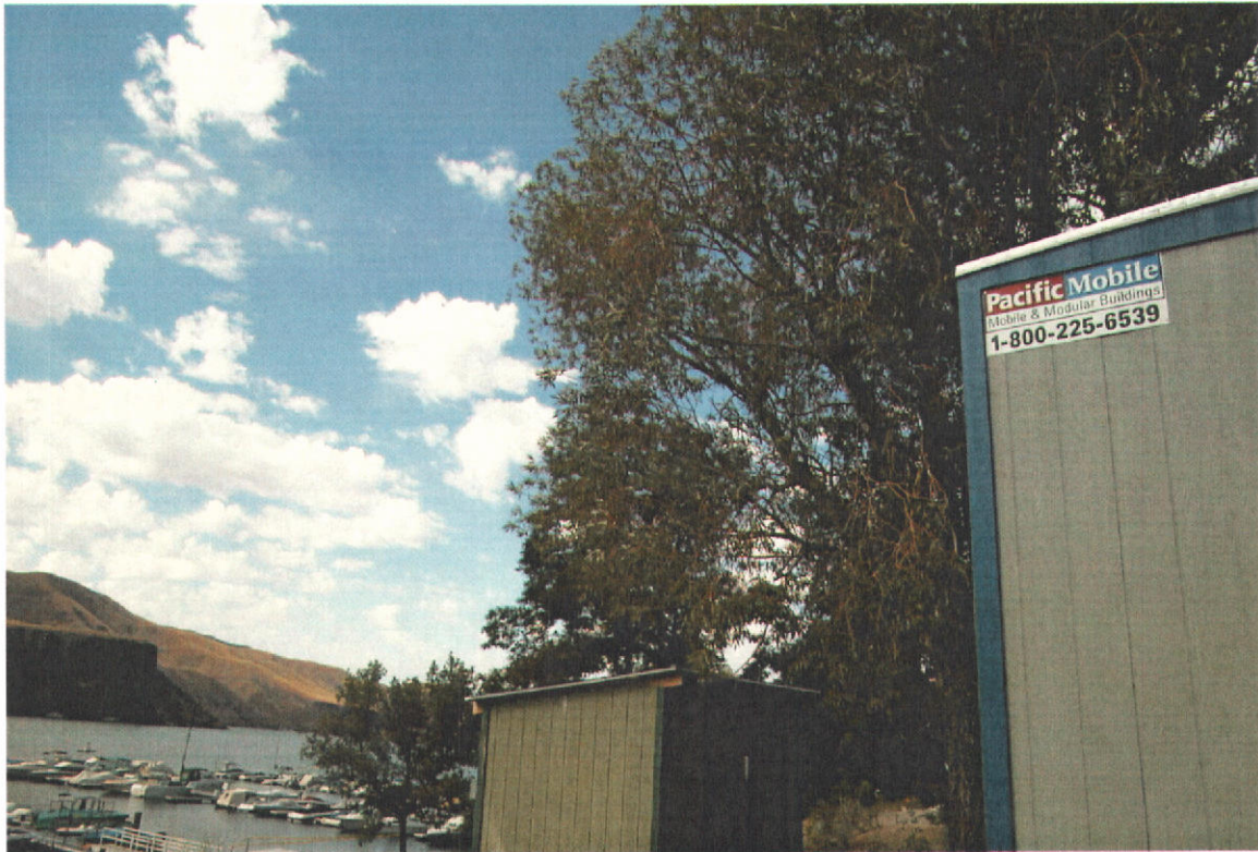
Well house is small building on left.
