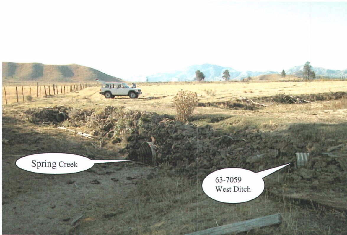
Photo 1. FX Oct. 4, 2001. Photos by RDH. POD view to south, plastic, rock dam. Culvert on right is for 63-07059. T02N, R07E, S04, NESESE.
