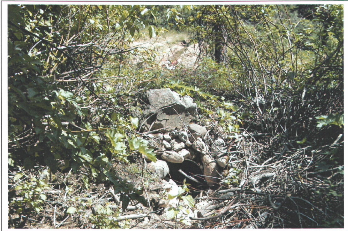
Photo 2. Culvert from above POD to ditch.
