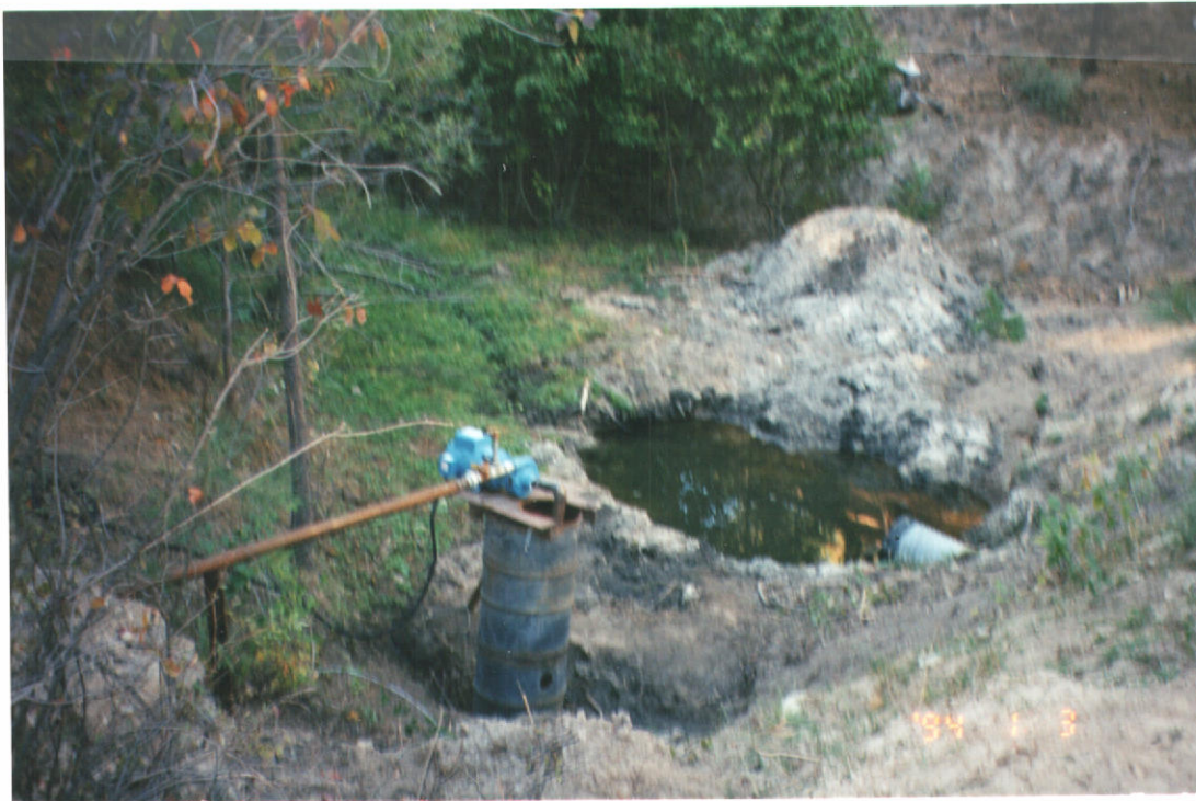
PHOTO # 1 LOWER POINT OF DIVERSION
