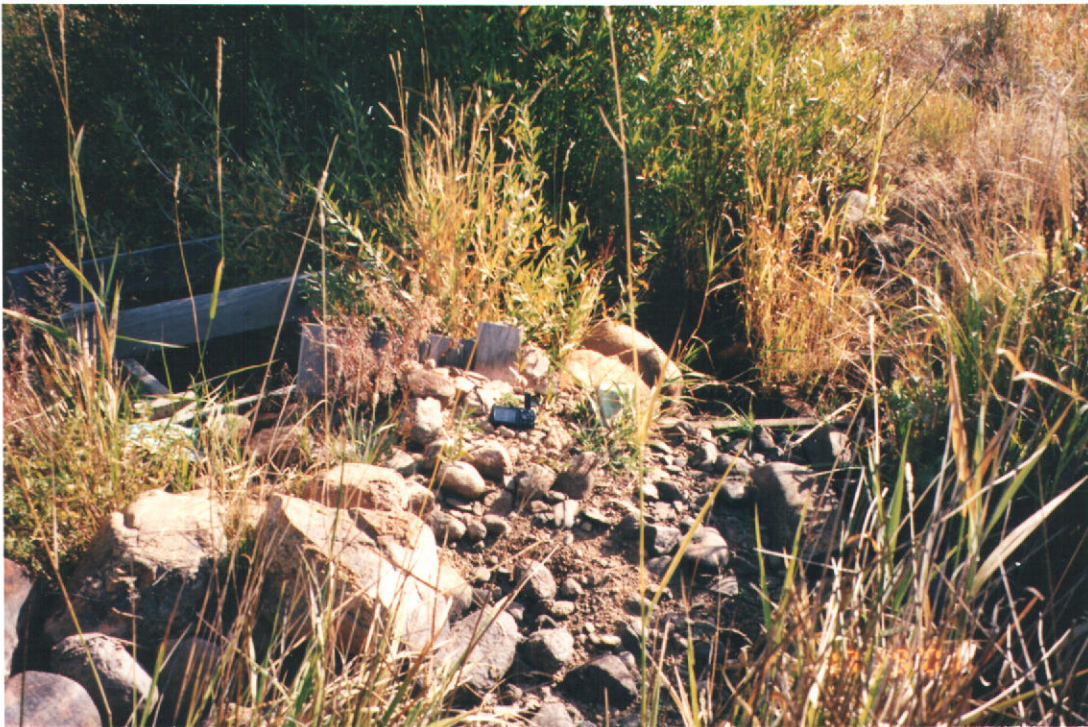
PHOTO #1 POINT OF DIVERSION ON TRAIL CREEK
