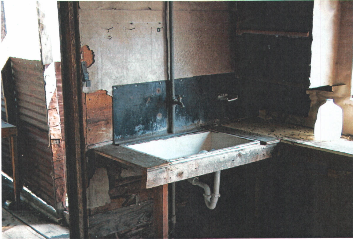
Photo 13: Inside cabin water piping into sink. Behind the sink wall is a shower outlet.
