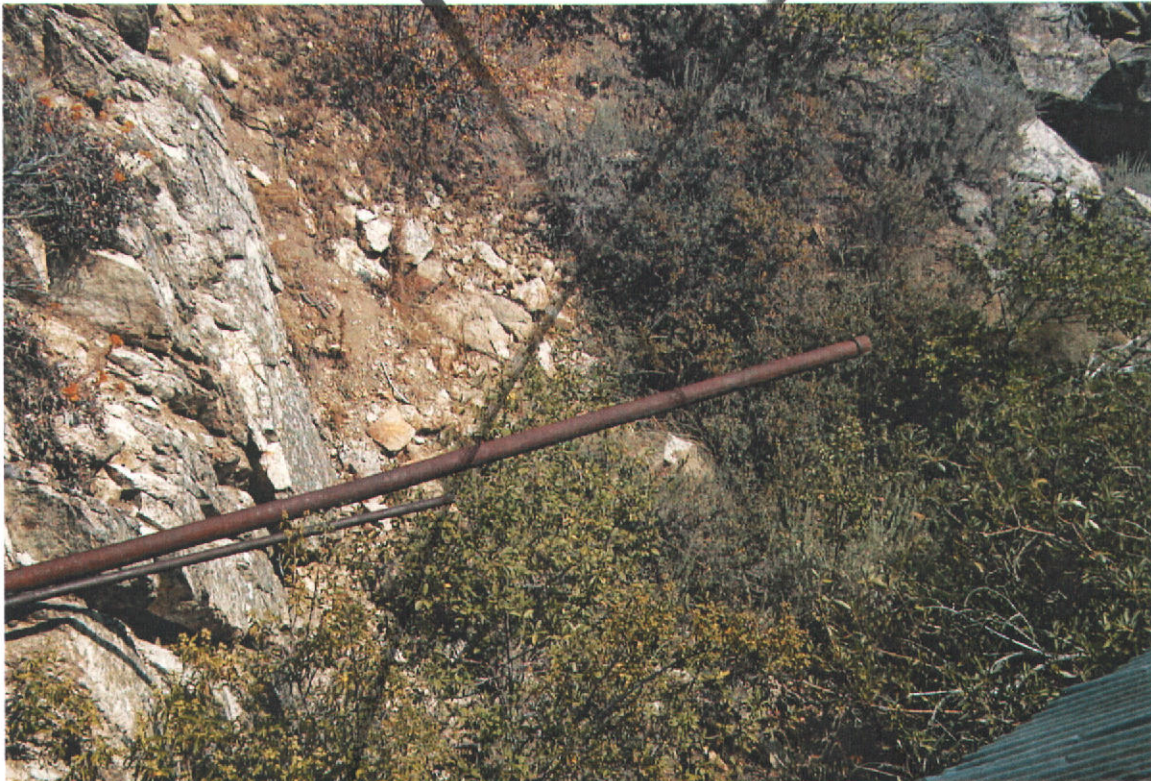
Photo 5: Main pipe line that went into wood tank next to Mill. Located in the SENW, S13, T03N, R03E.
