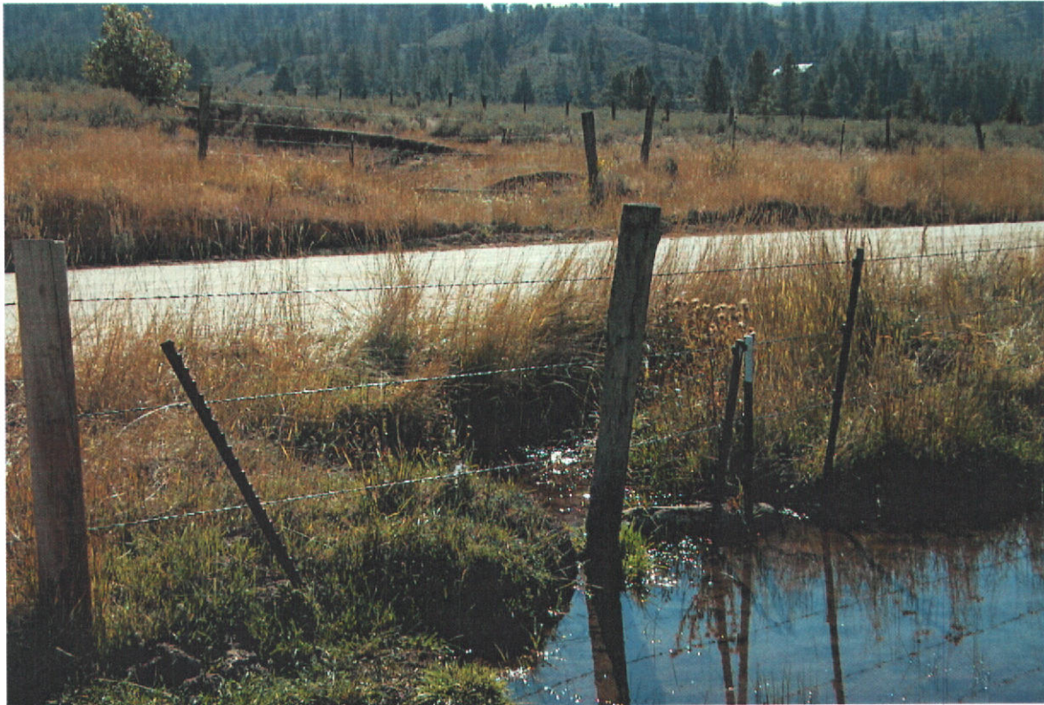
Photo 3. Photos by RDH. Ditch flows under county road.
