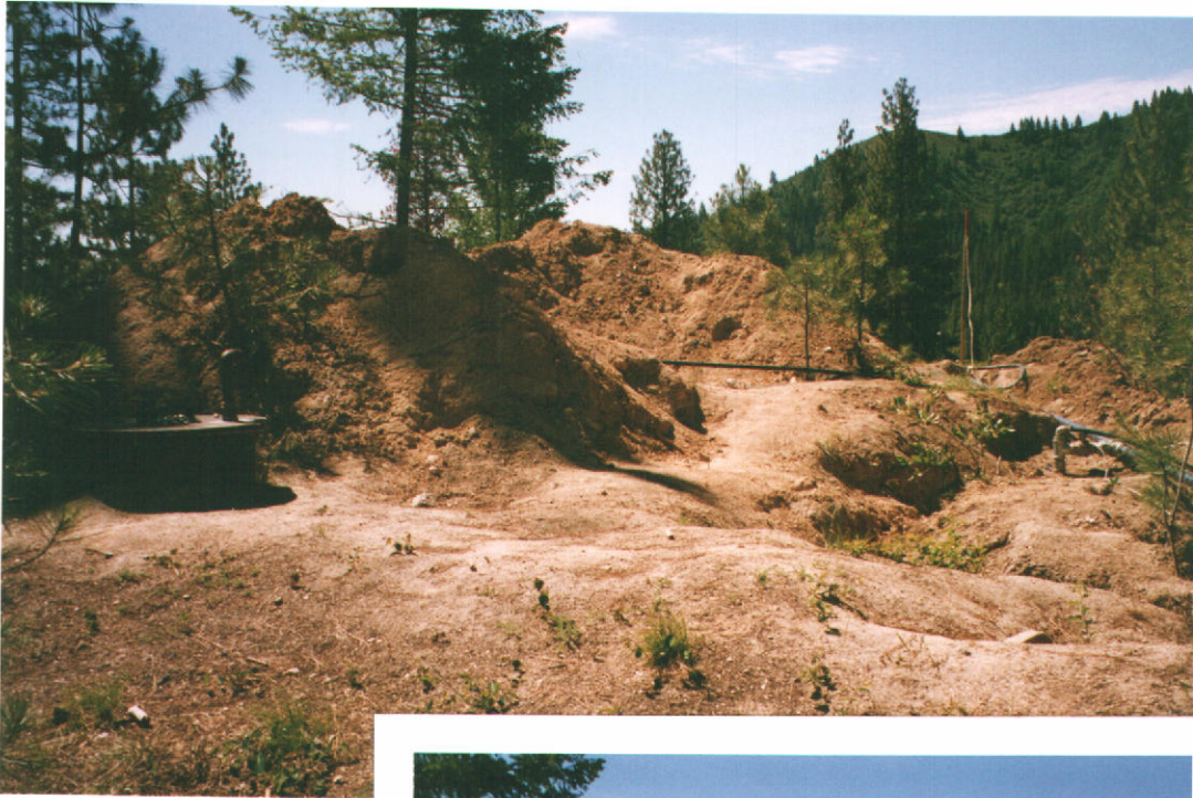
PHOTO #3 STORAGE TANK SITE
