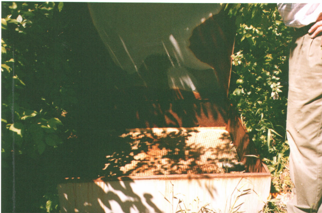
PHOTO #2 EXISTING COLLECTION BOX AT LOWER SPRING
