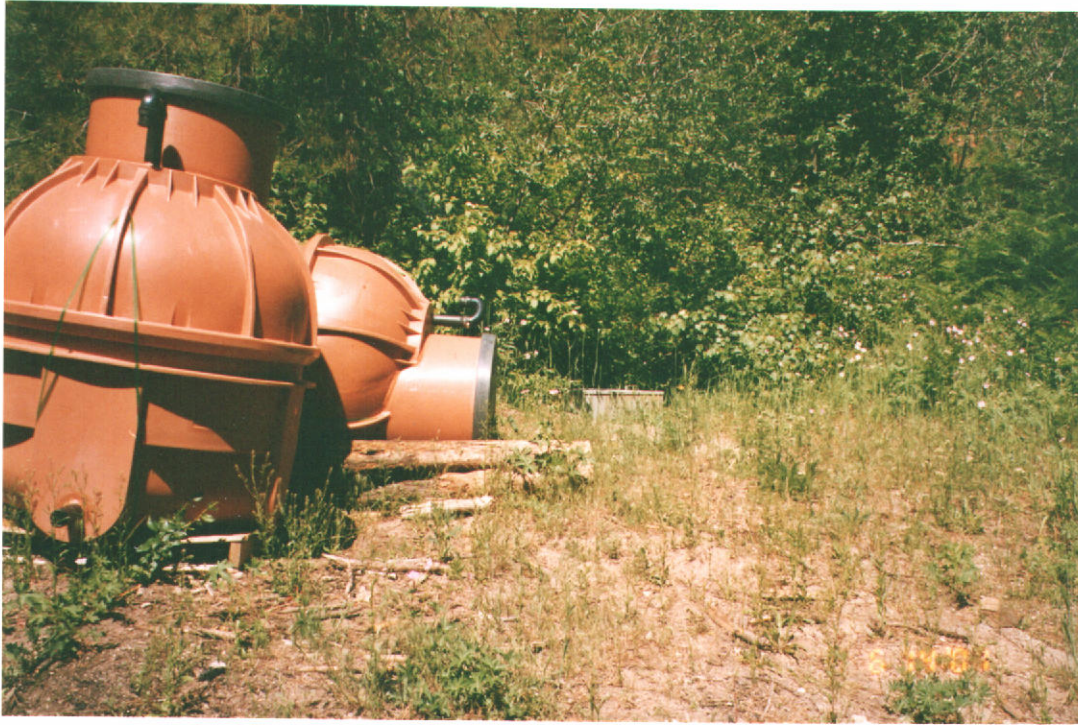
PHOTO #1 POD AT LOWER SPRING AND NEW COLLECTION BOXES TO BE INSTALLED
