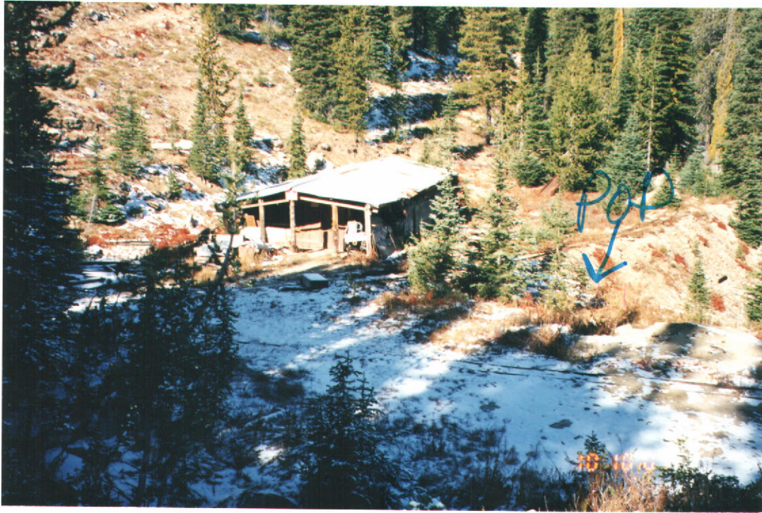
PHOTO #3 POD FOR THE MILLING OPERATION LOOKING WEST FROM THE ROAD
