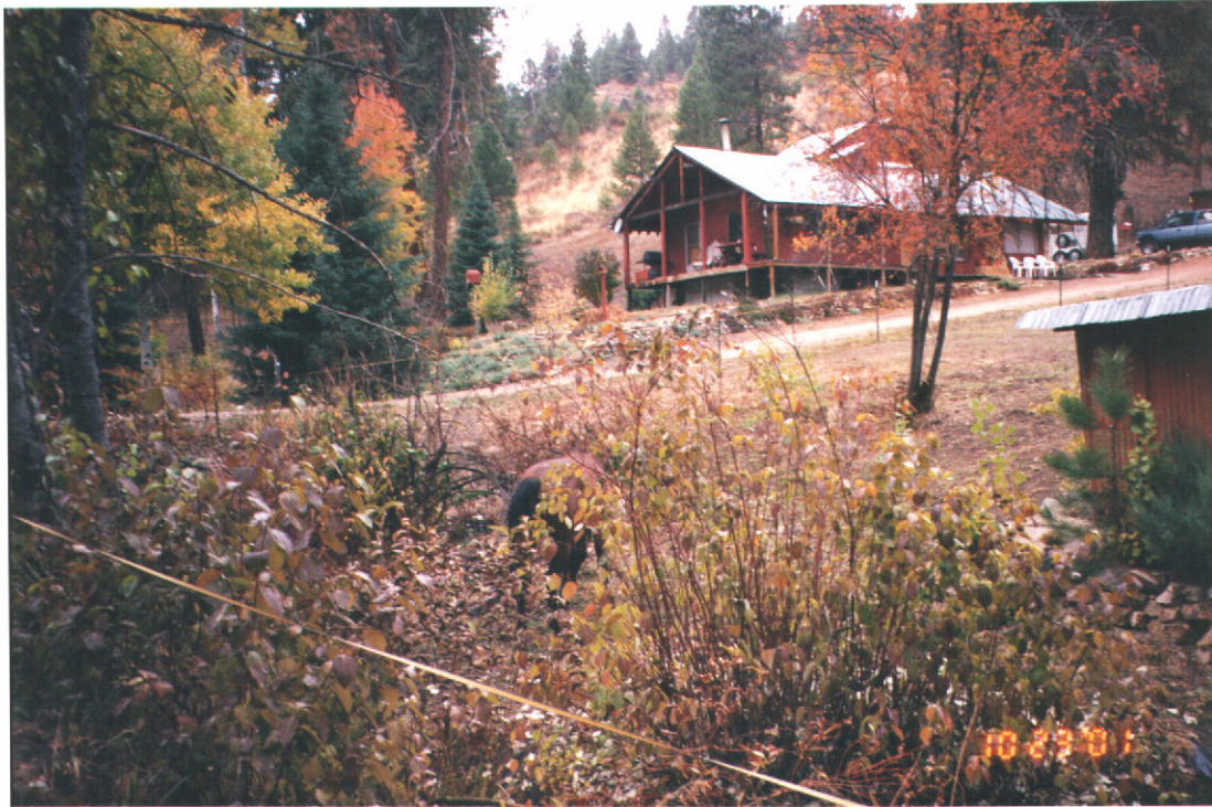
PHOTO #3 PART OF THE PLACE OF USE LOOKING NORTH- WEST FROM THE ROAD
