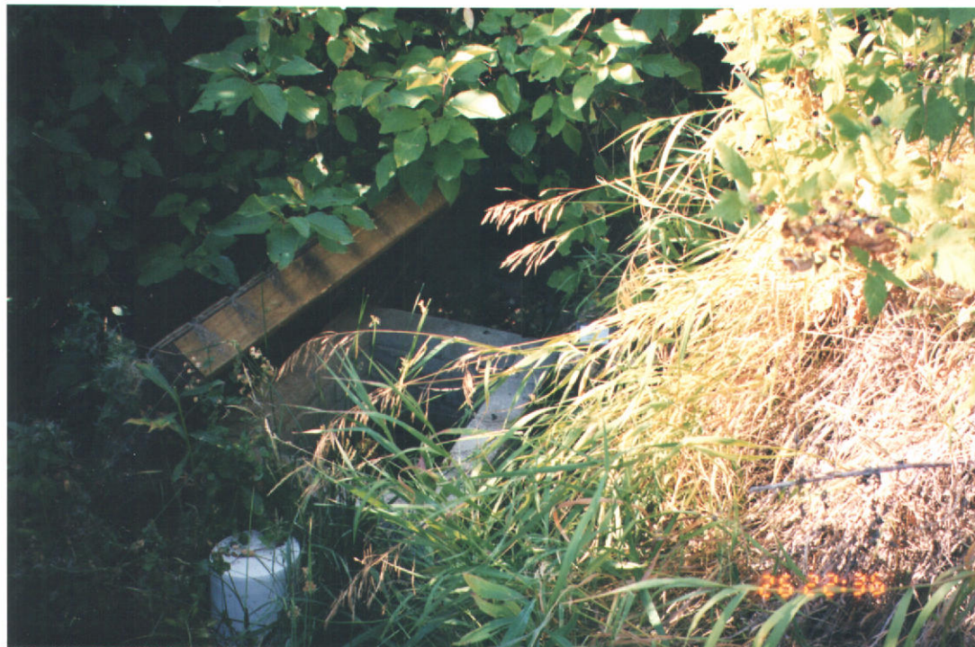
PHOTO #1 SPRING BOX AT POD
