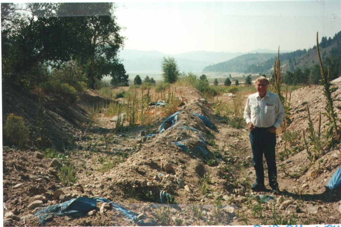
Dirt diversion on Bird creek. Creek on left, ditch on right.
