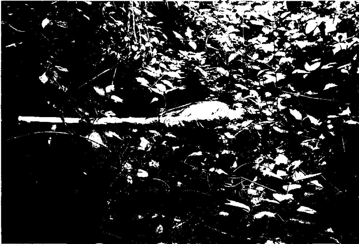
Photo 1. FX Aug. 20, 2001. Photos by RDH. 63-4225; Upper POD from Trail Creek, Located in T01N, R07E, S09, NENE. Eight inch PVC pipe from POD.
