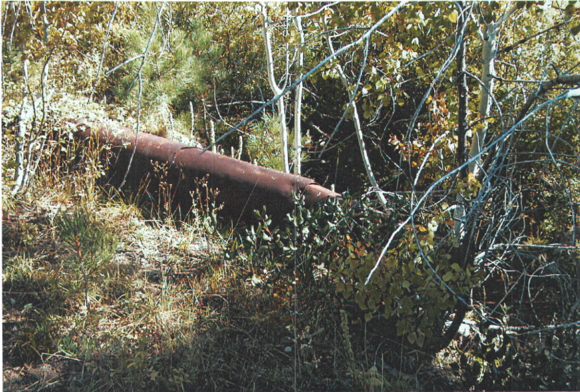
Photo 2. Photos by RDH. Photo of 14-inch culvert used when pool is backed up from POD then flows into ditch.
