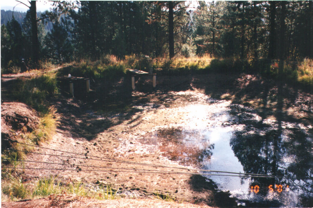
PHOTO # 7 SMALL POND ABOVE THE TOWN. (IT WAS BEING REPAIRED ON 10/05/2001
