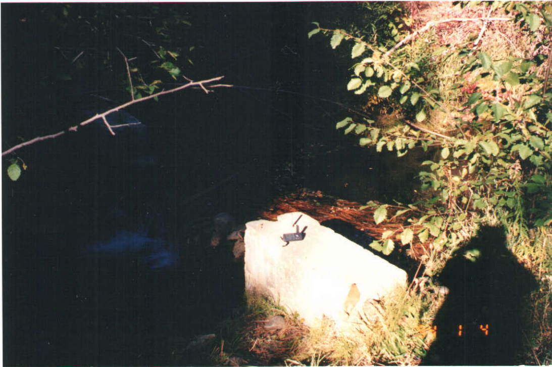
PHOTO # 1 POINT OF DIVERSION
