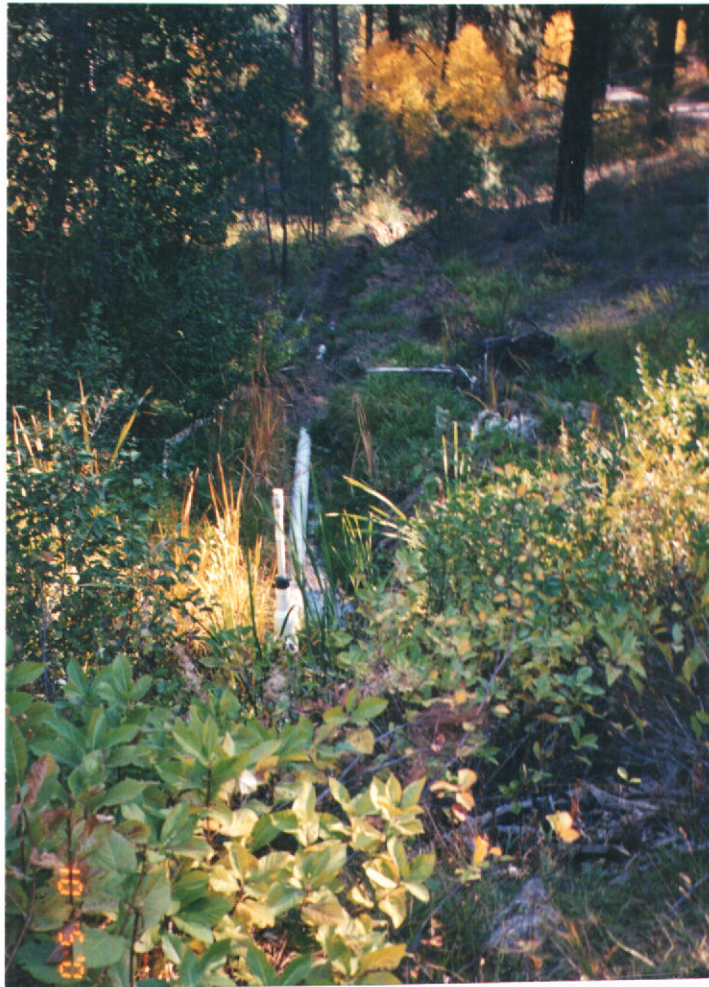
PHOTO # 5 PIPES BELOW THE UPPER POND LOOKING DOWN FROM THE DAM
