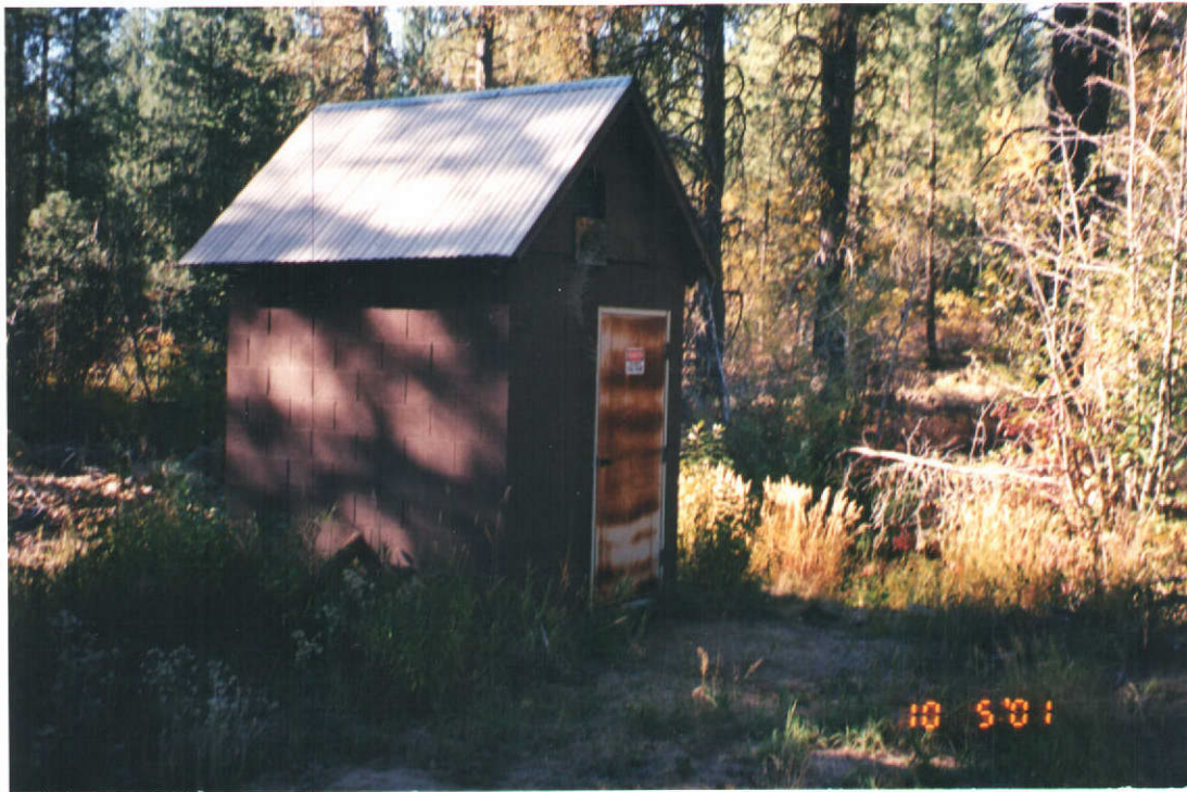
PHOTO #2 PUMP HOUSE AT THE POINT OF DIVERSION
