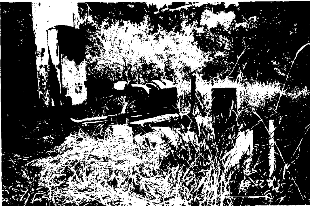
PHOTO #2 PUMP & MOTOR AT THE POD
